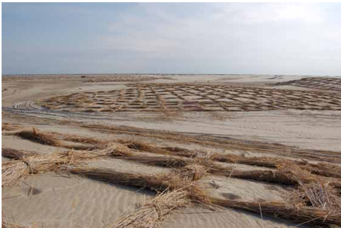
Fig. 53: Mechanical fixation of sand sheets and dunes with reed cane
