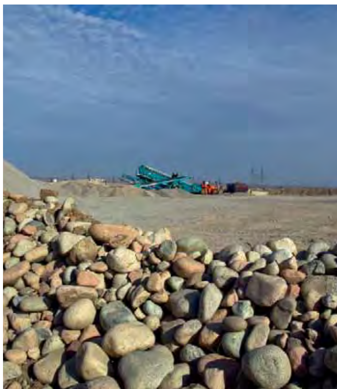
Construction of the Western Europe-Western China Highway close to the Aspara Basin.
