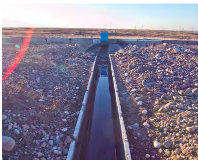
A segment of irrigation network.
