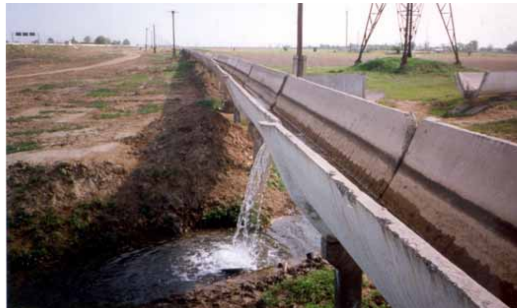
Concrete canalettes leak badly, in this case for unauthorised access - Syrdariya, Uzbekistan
