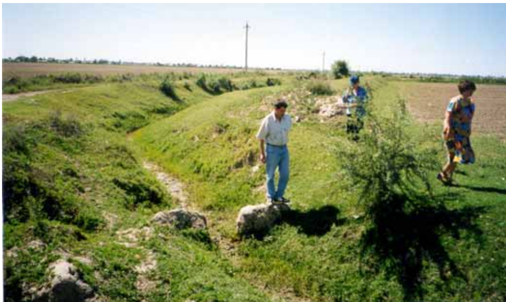
Farm supply canals and control structures are poorly maintained - Farm 03, S Kazakhstan
