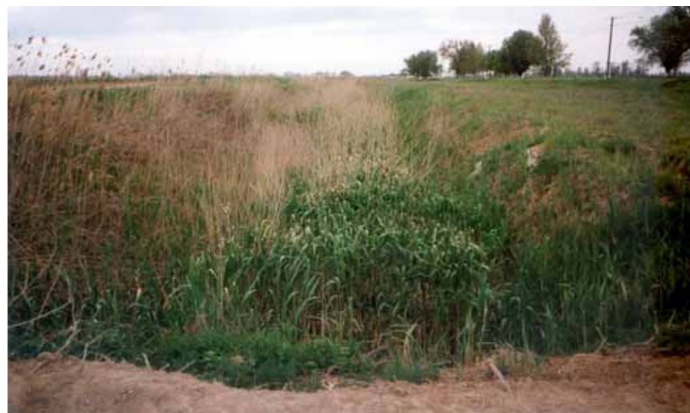
Farm drainage collectors are silted and weedy so that water backs-up into field drains - Farm 22, Surkhandariya
