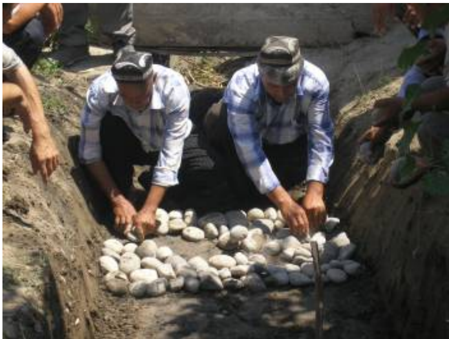
Figure 1.8. Placing riprap beneath the foundation of a water-measuring device.
