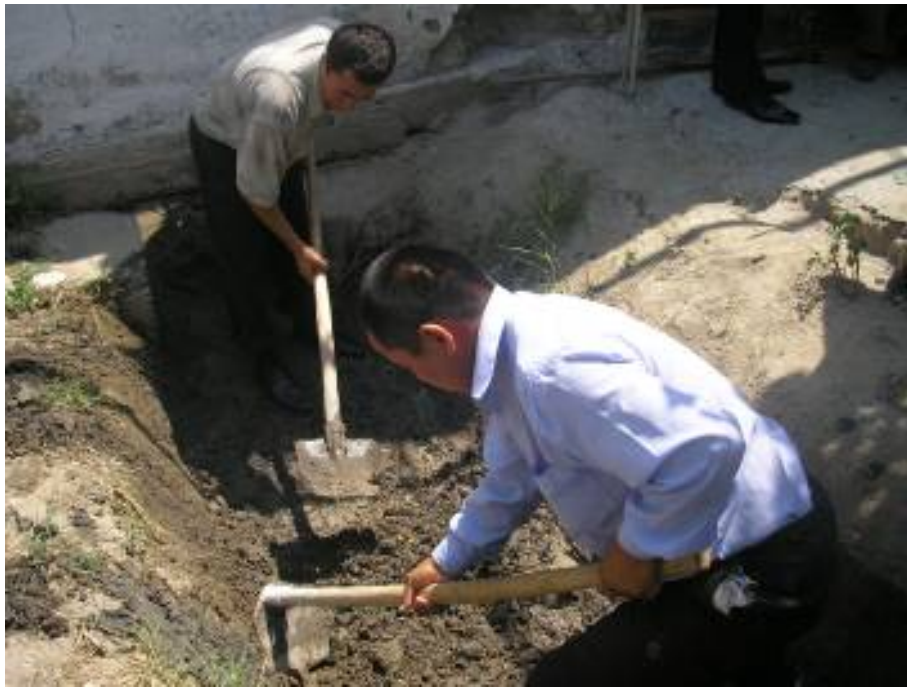
Figure 1.7. Cleaning the canal bed from silts and aquatic vegetation.
