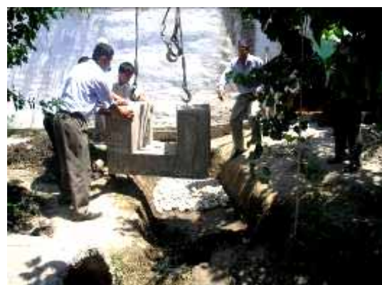
b) Assembling pre-cast flumes
