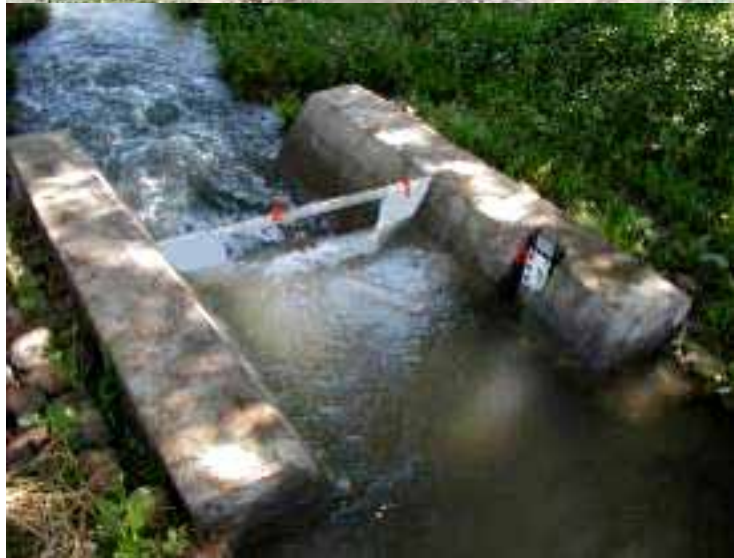
Figure 5.3 Gauging posts equipped with Chipoletti weirs: where: 1 – Chipoletti weir; 2 – stiffening bar; 3 –gauging rod “RUG”
