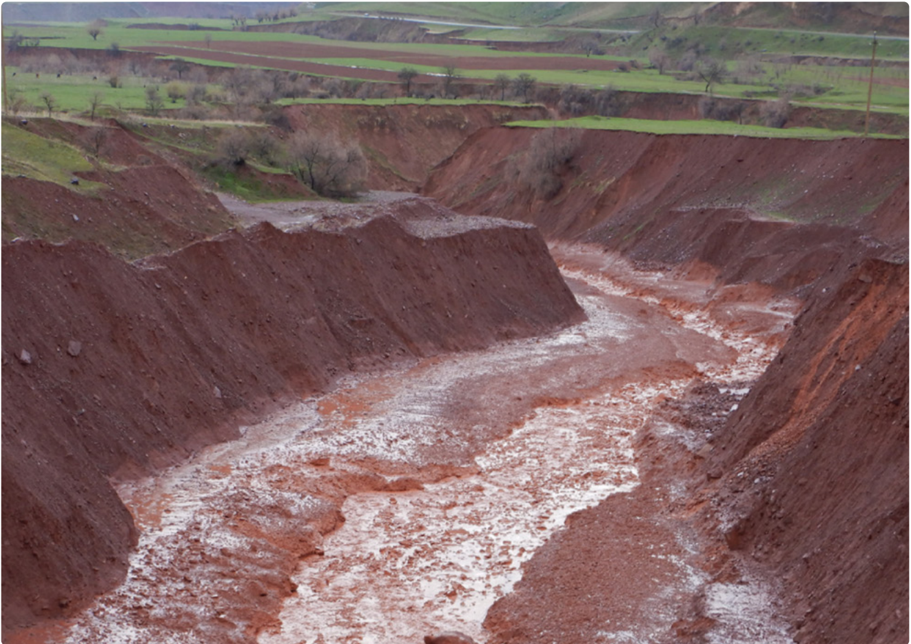
Figure 5: Streambank Erosion along a Vakhsh River Tributary Transporting High Sediment Load, Following a Low-Intensity Storm
