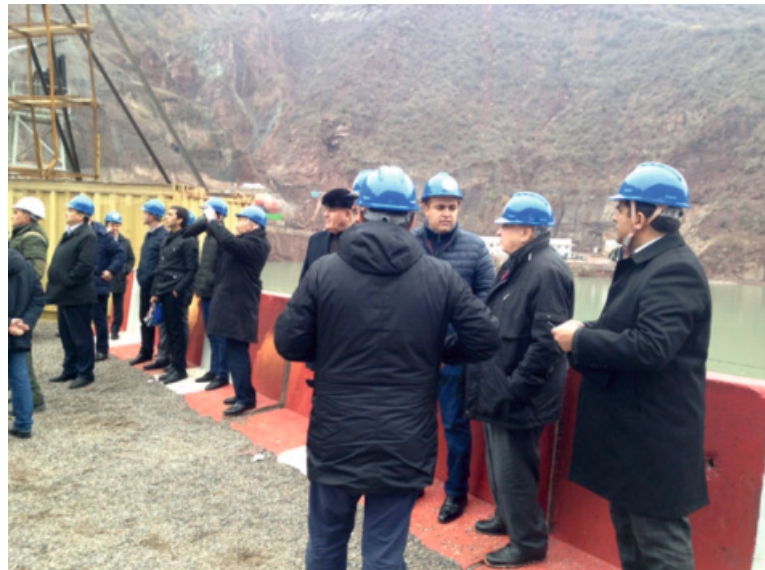
On the right, headwater created by temporary dam and the construction site, which will be flooded in the future
