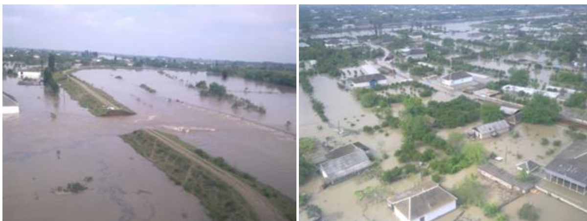
Figure 5 – Kura flooded several administrative regions in 2010 year in Azerbaijan.
