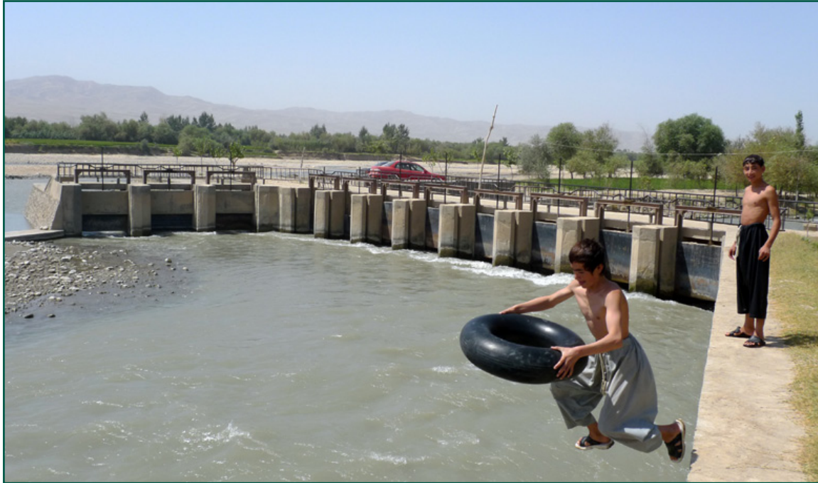
Image 2: Sharawan headwork (right, eight gates) and Sharan spillway (left, three gates)
