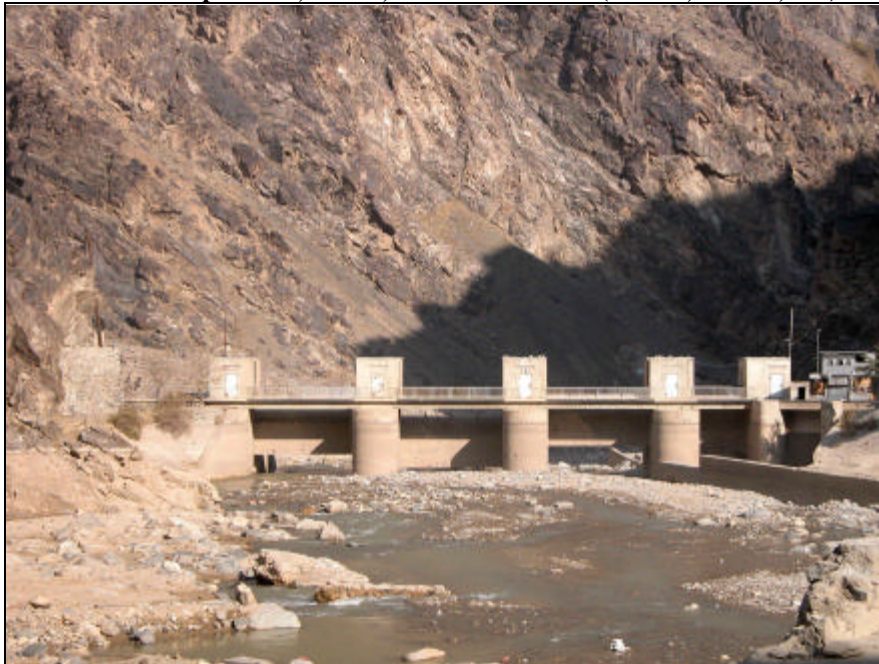
Picture 73 Band-i Mahipar dam, Kabul, 5 December 2003 (N34.56, E69.48, NE)
