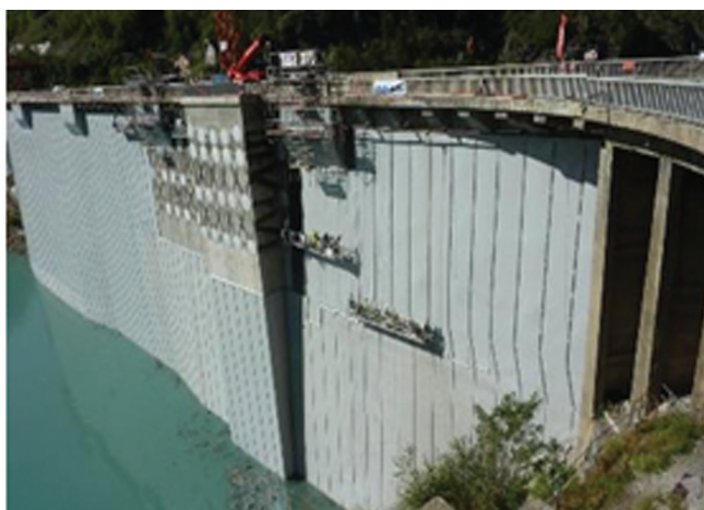
Fig.1. Installation of the SIBELON® geomembrane system at Chambon dam
