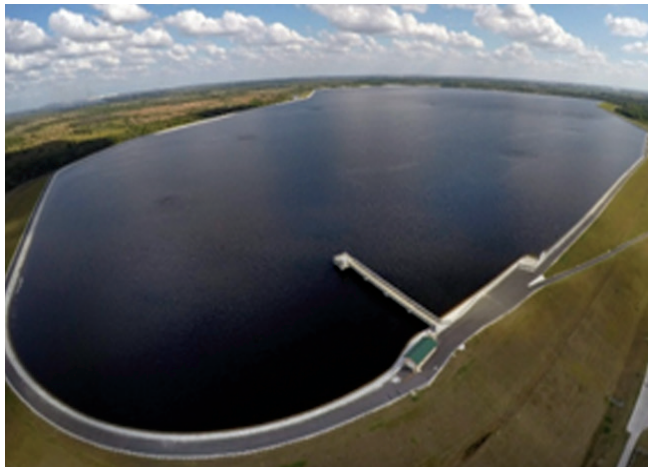
Fig.5. C.W. Bill Young reservoir in operation after rehabilitation, which included placement of a covered SIBELON® geomembrane system
