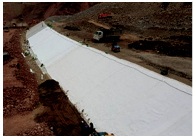
Fig.4. Installation of the SIBELON ® geomembrane system in the Rogun upstream cofferdam
