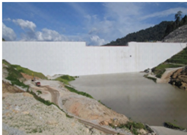
Fig.2. View of Susu dam during impoundment
