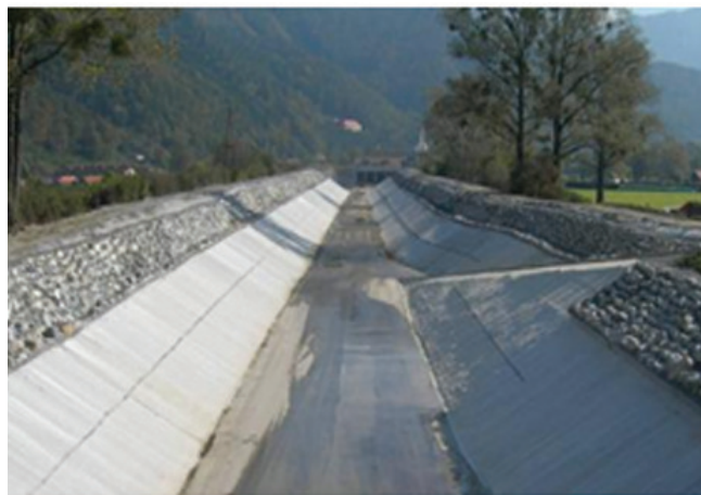
Fig.7. Pernegg canal after completion of the waterproofing works
