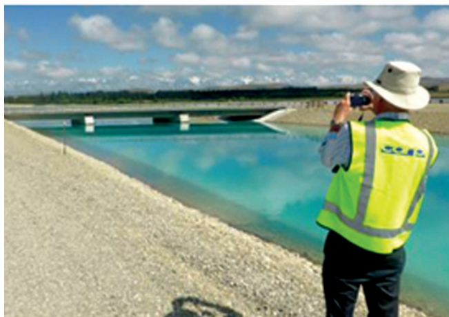
Fig.8. Tekapo canal after completion of the remedial works
