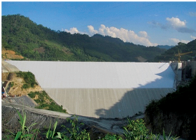
Fig.3. Nam OU VI rockfill dam after completion of the second stage installation of the exposed SIBELON ® geomembrane system
